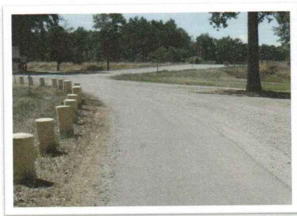
Existing Asphalt Trail
