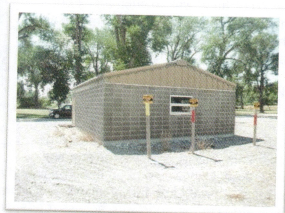
Williston Basin Pipeline Building
