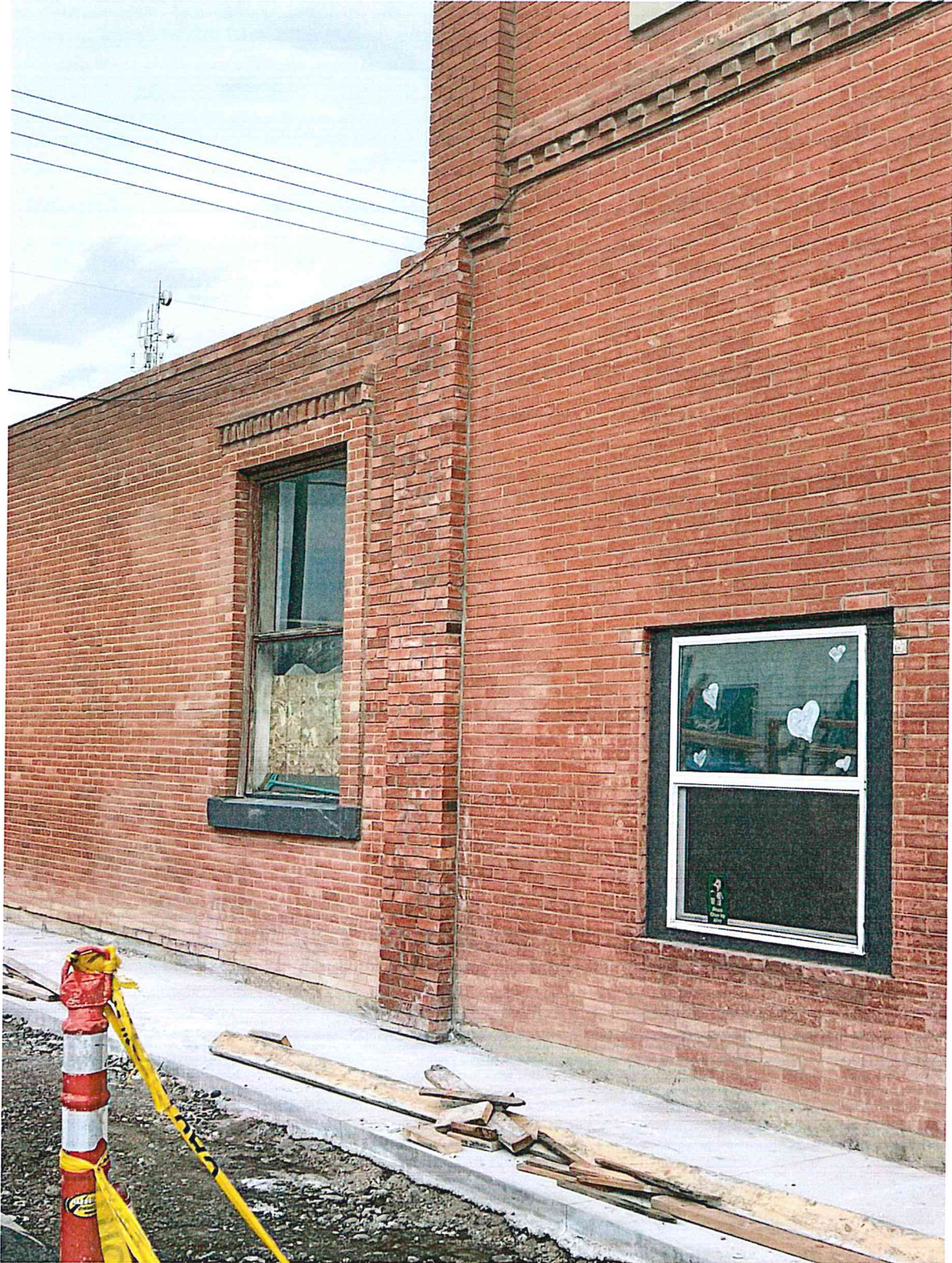
Seam between main building and garage repaired:
