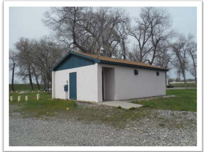
Existing Public Restroom Building
