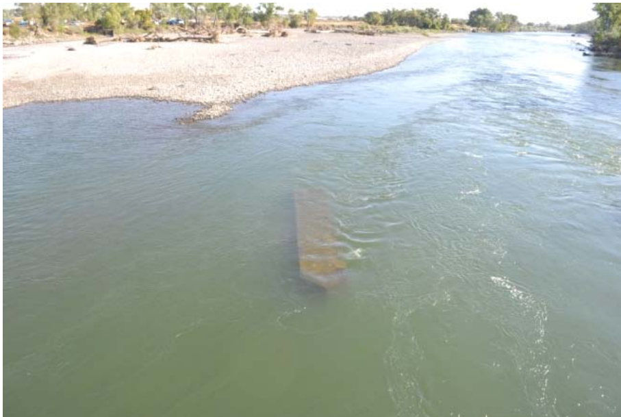
Figure 1: Current WTP intake structure, looking downstream from the highway bridge
