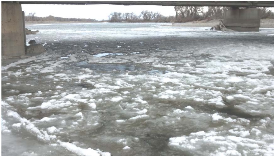
Figure 5: Frazil ice beneath highway and railroad bridges, December 2012
