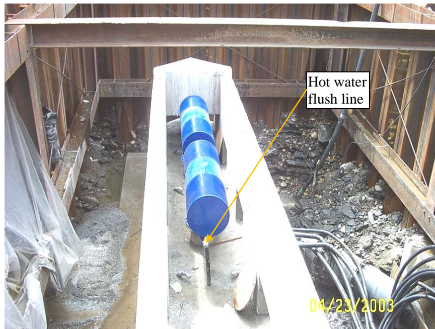
Figure 12: Picture of current intake during construction showing hot water flush line
