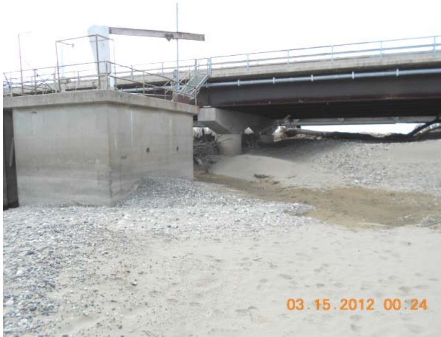
Figure 2: Historic intake structure and sediment deposition, looking upstream at highway bridge
