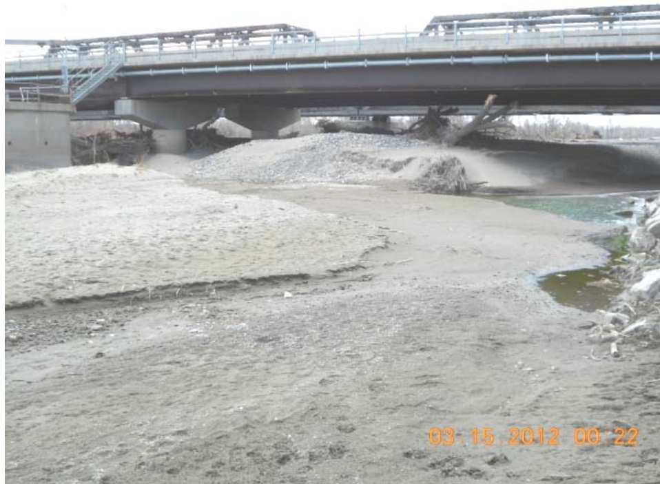
Figure 13: Sediment deposition beneath railroad and highway bridges. Looking upstream.
