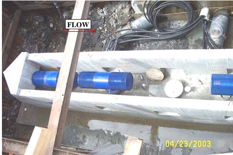
Figure 4: Photo of current intake during construction, showing screens
