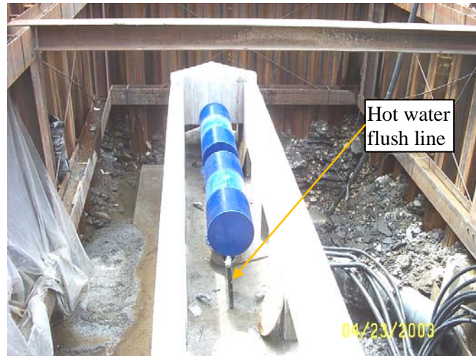
Figure 27: Picture of existing intake during construction showing hot water flush line
