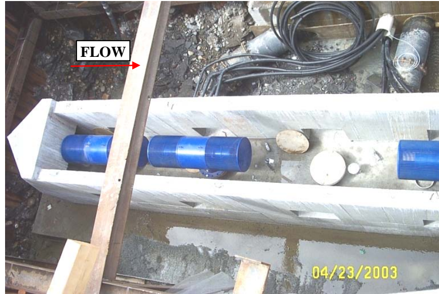
Figure 4: Photo of existing intake during construction, showing screens
