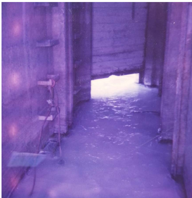
Figure 52: Inside chamber of historic intake, frozen solid, 12/21/1998
