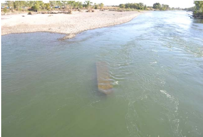
Figure 1: Existing (new) WTP intake structure, looking downstream from the highway bridge
